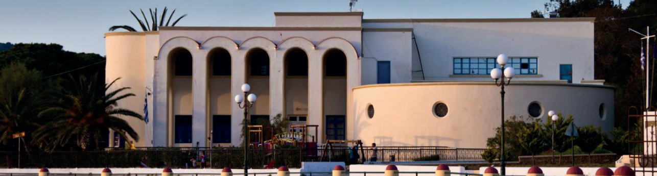
Primary School built in the Italian Fascist style of Razionalismo, Lakki, Leros Island, Dodecanese Islands, Greece ©ATRIUM
