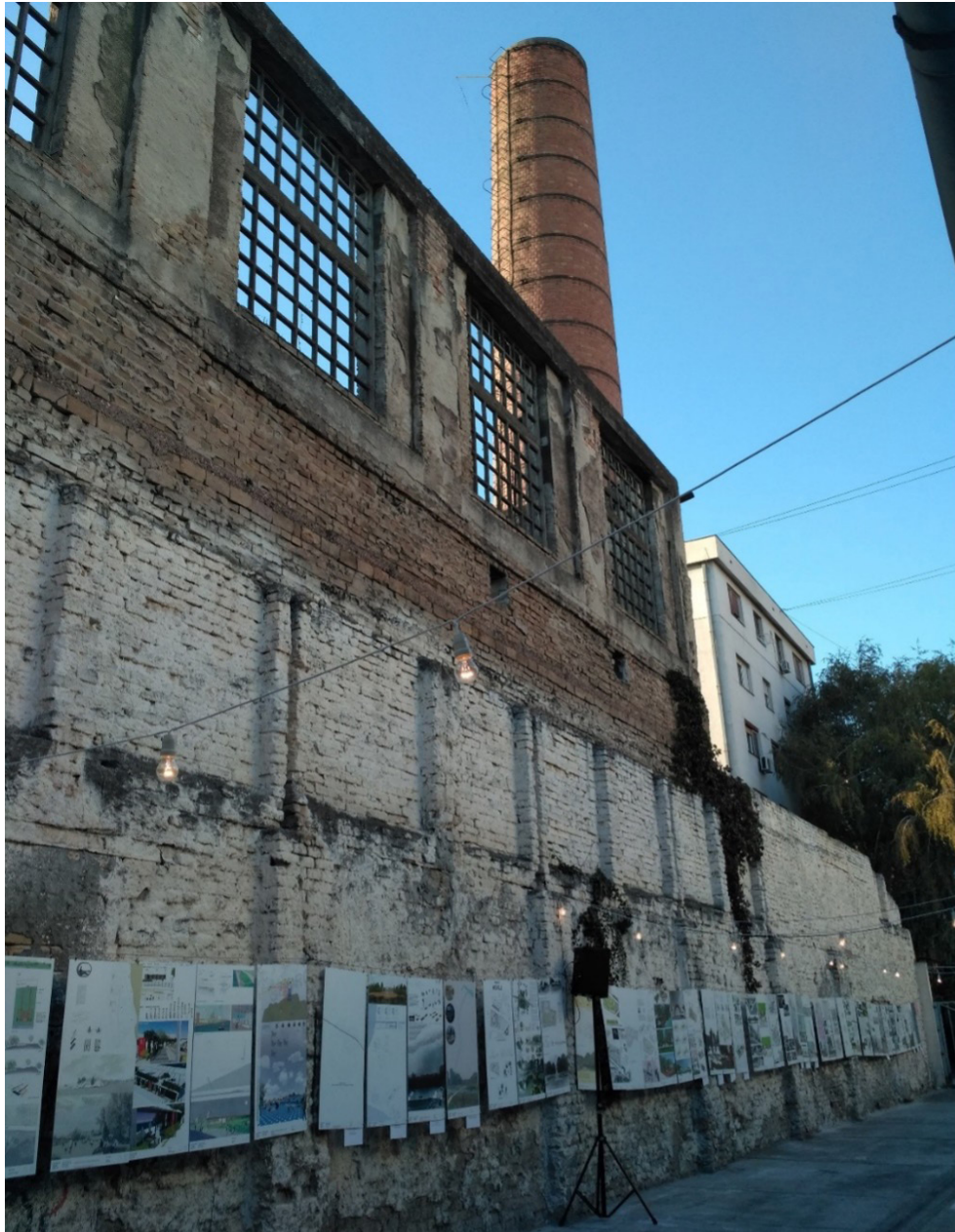
Silk factory before renovation, September 2017. Photo: Jasmina Kočovska
